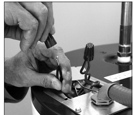
Figure 19 - Connecting the electrical wires.
